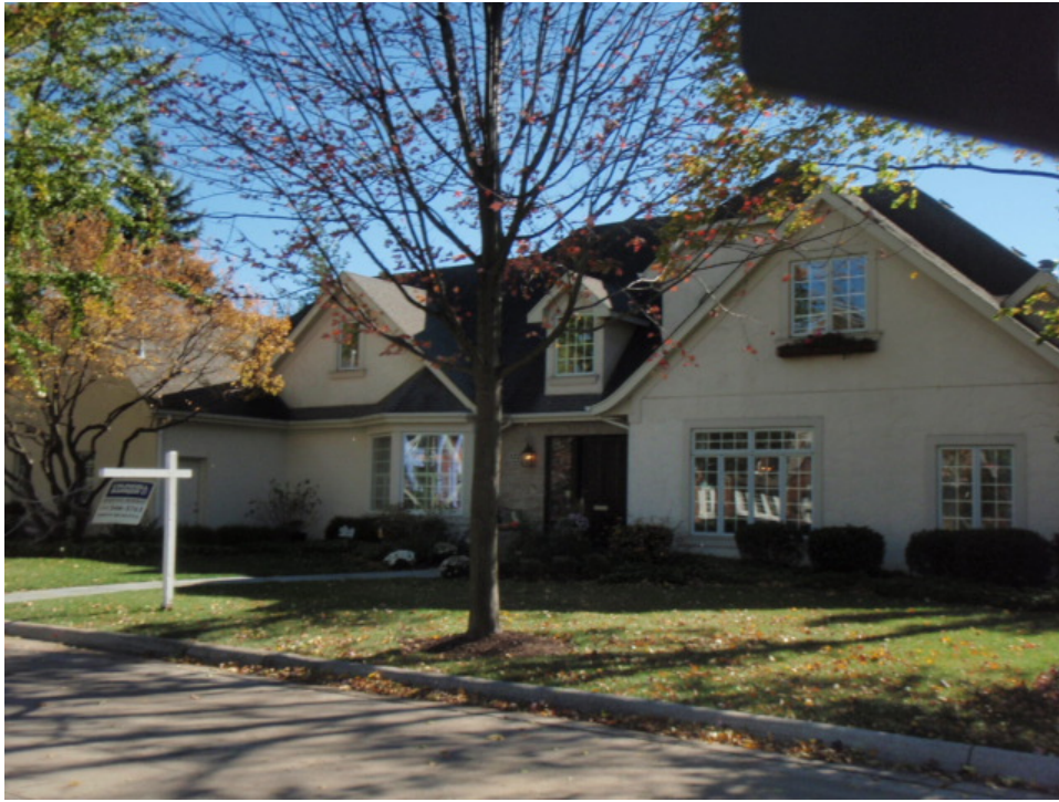
Photo 1. This is the front (north elevation).
